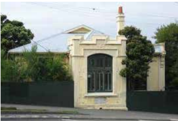
The Crèche, Buckle Street
