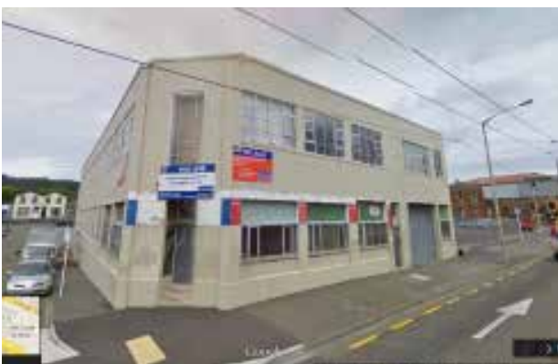
SIS Building, Taranaki Street
